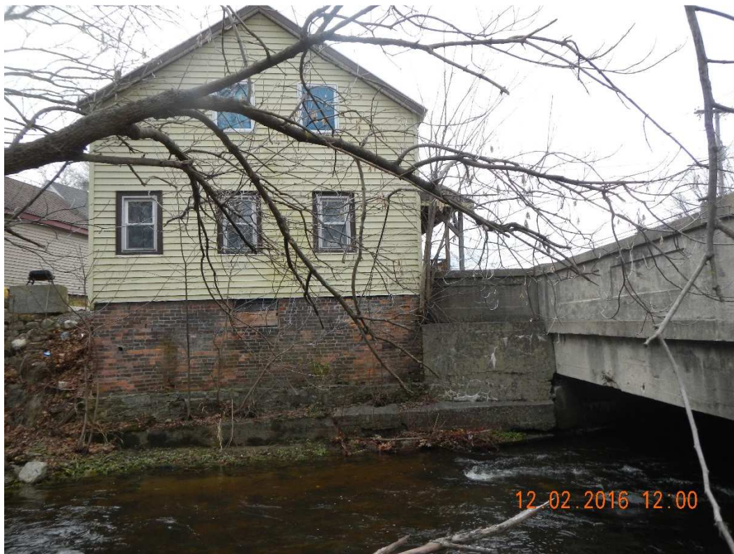
Figure 3: Structure Foundation in Contact with Bridge
