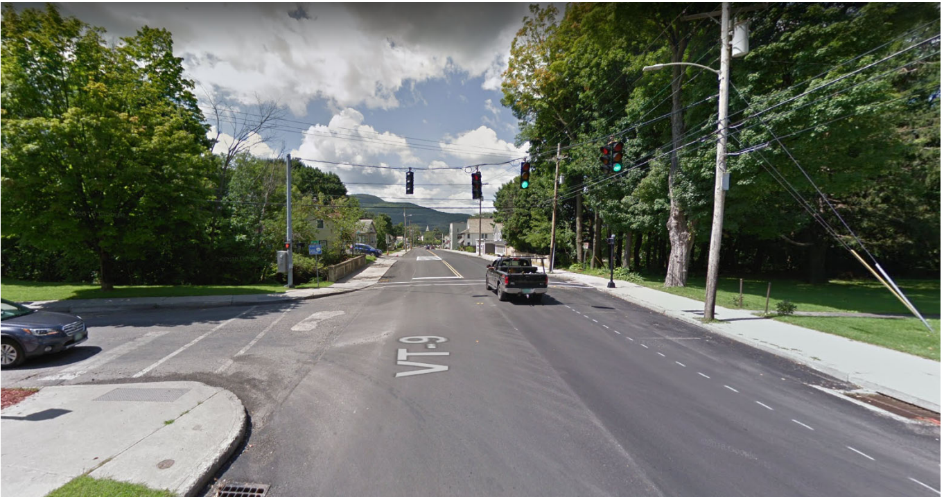
Picture 1: Looking West Over Bridge
