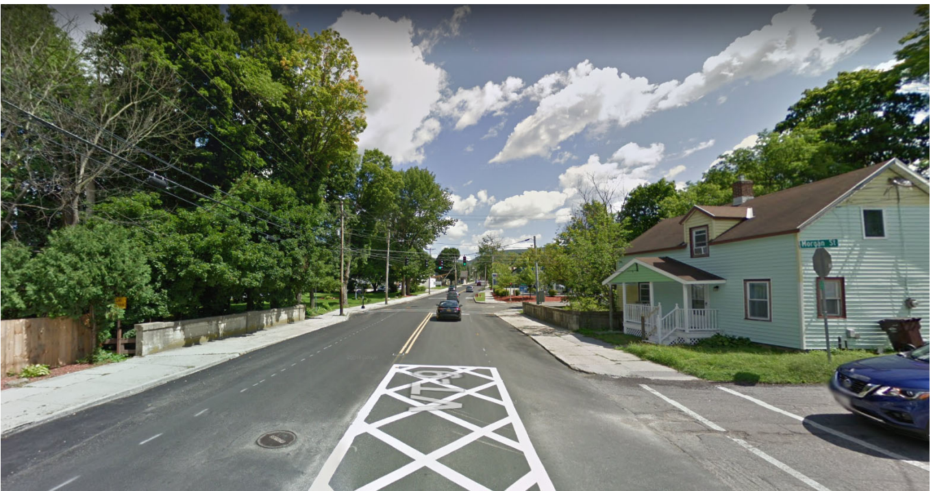
Picture 2: Looking East Over Bridge
