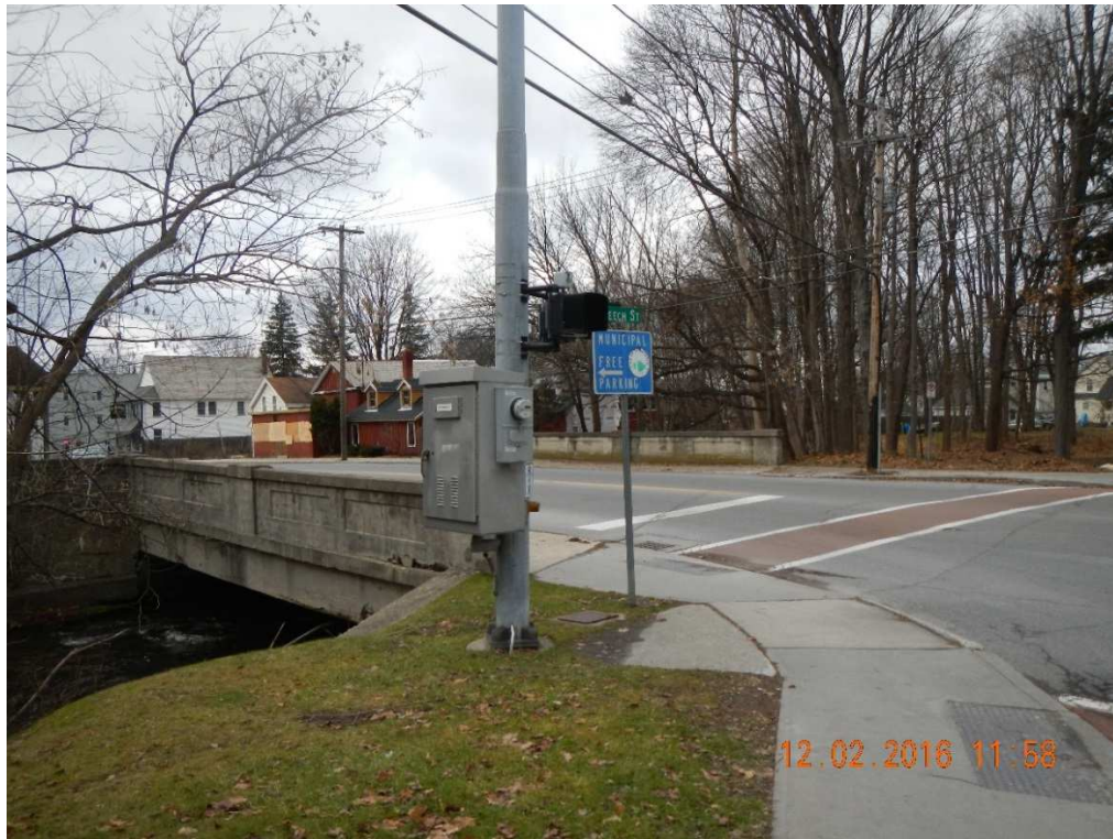
Figure 4: Utility Lines Above and Parallel to Bridge
