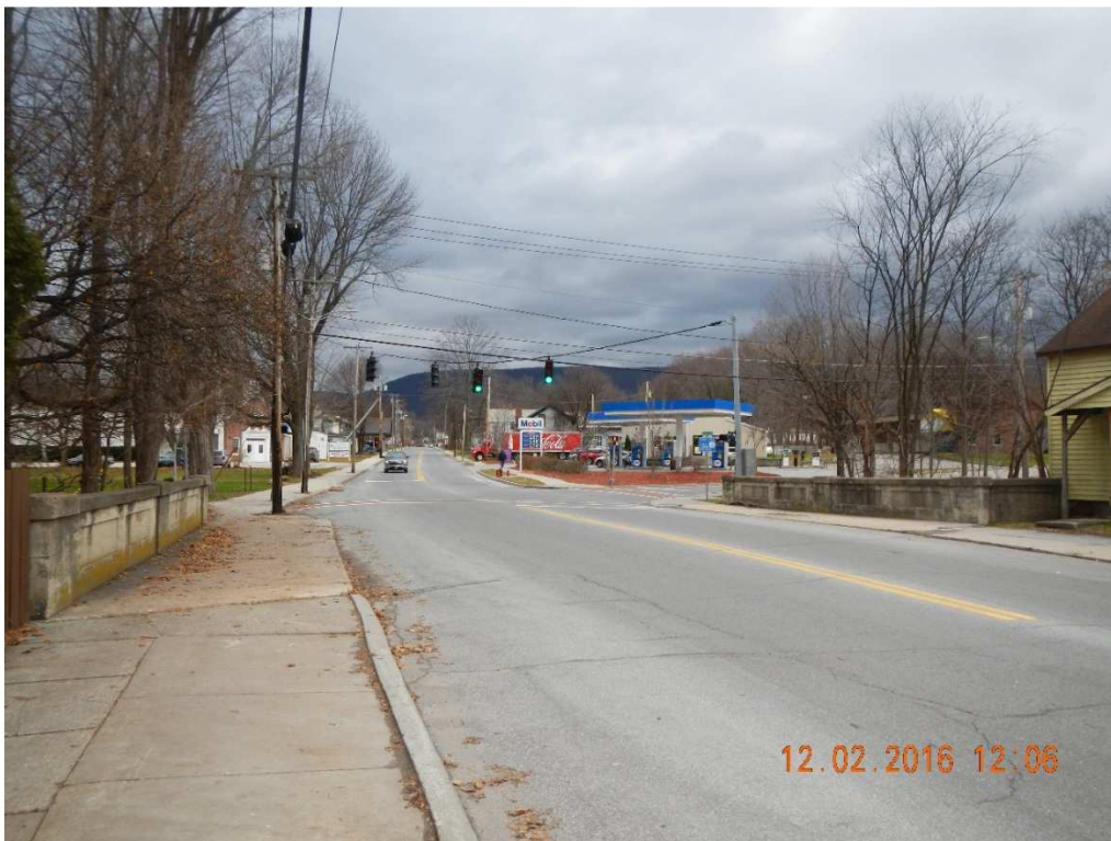
Figure 5: Looking East Over the Bridge
