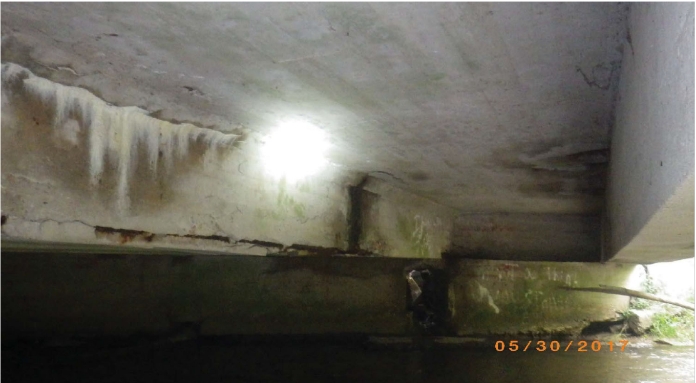
Picture 5: Beam and Abutment Deterioration
