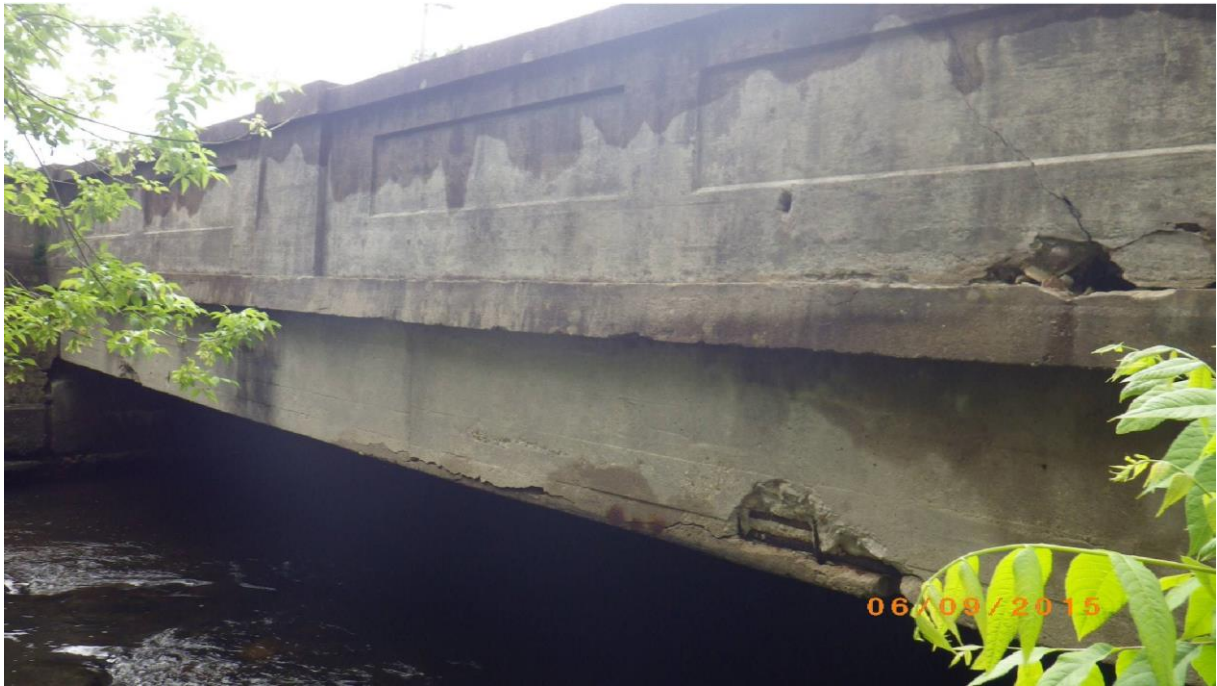
Figure 2. Bridge No. 6 Beam and Rail
