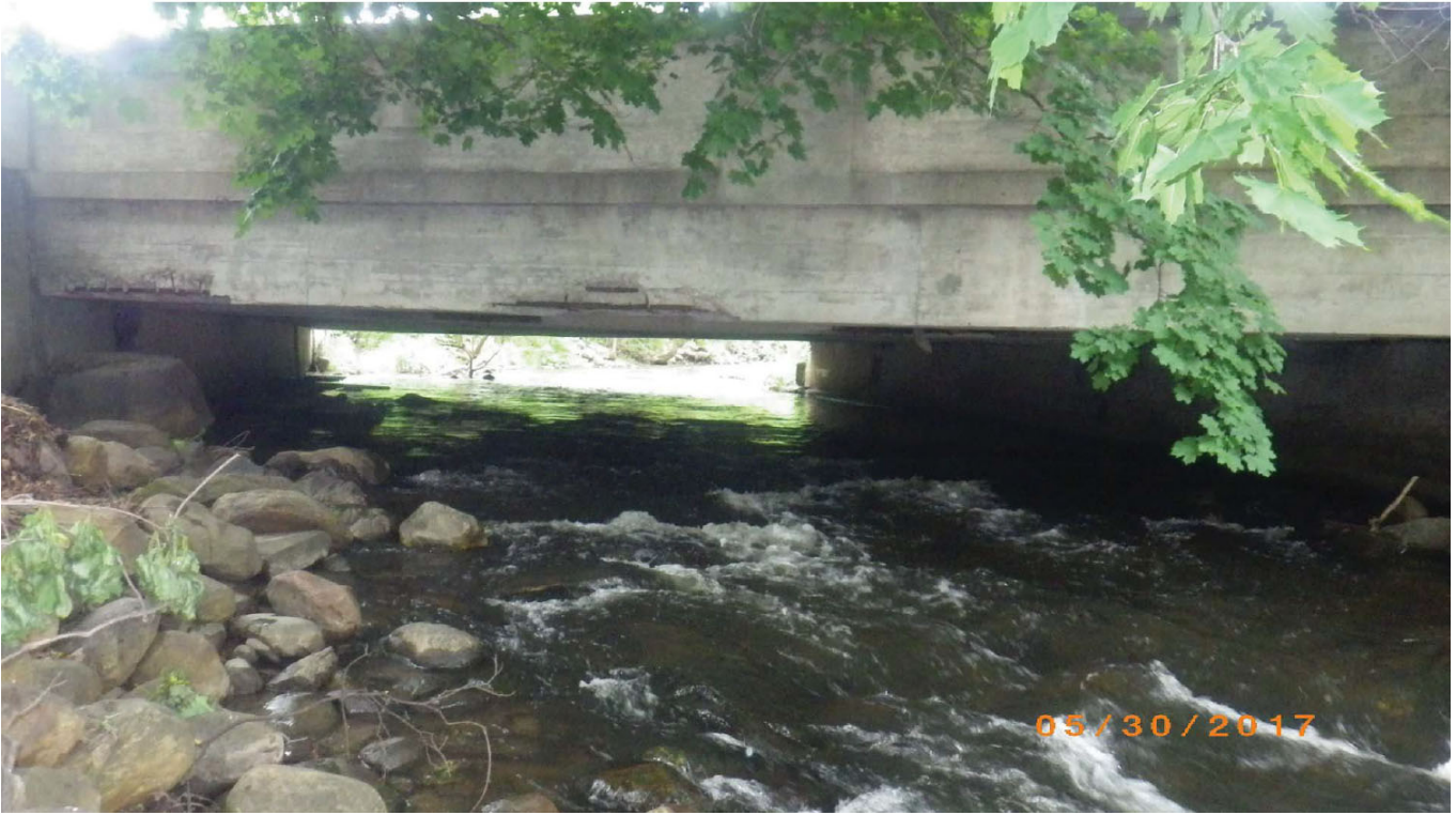
Picture 3: Looking at Upstream Fascia
