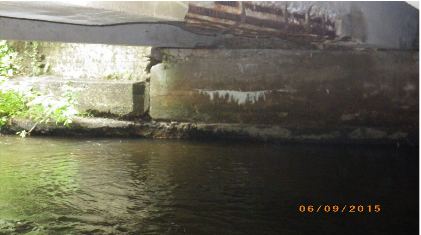
Picture 4: Abutment Scour and Deterioration
