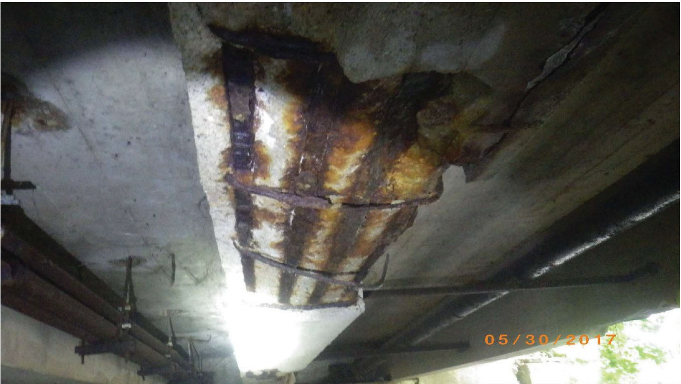
Picture 6: T-Beam Deterioration and Utilities
